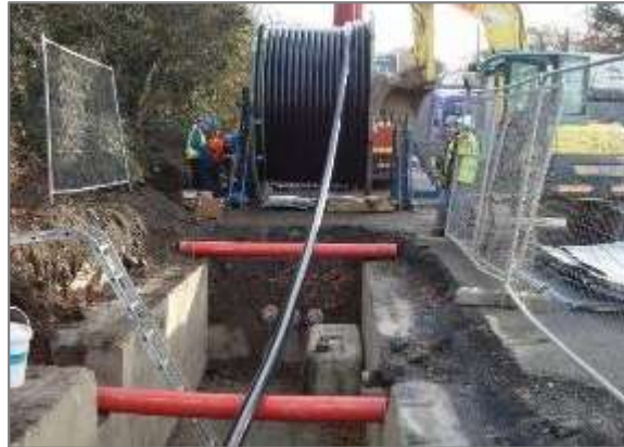
Figure 8 - HV cable pulling procedure (Drum set-up example)
